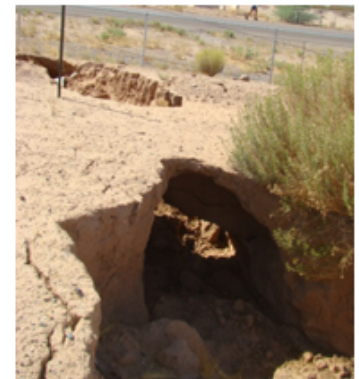
Fissure near freeway 202 & I-60
