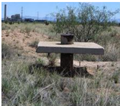
Displaced well pad.
