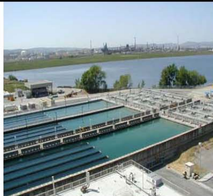
Drinking Water Treatment Plant
