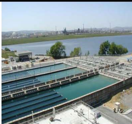
Drinking Water Treatment Plant
