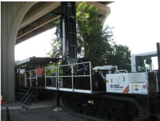
Field scientists pick the sonic technique because of the information you get from the high quality core. The sonic method greatly reduces the risk of project failure due to unknown or difficult subsurface conditions.
