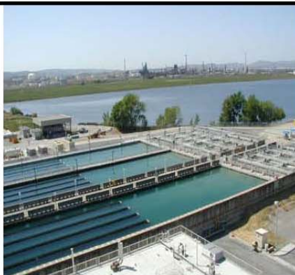
Drinking Water Treatment Plant
